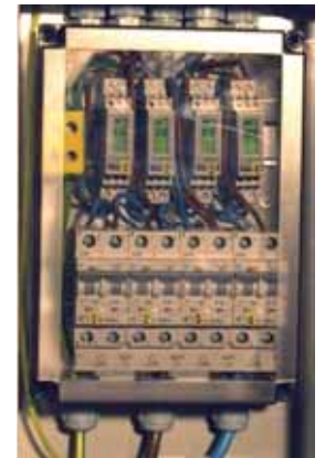
4x16A kbv. 4 x kwh IP66/67 kit
